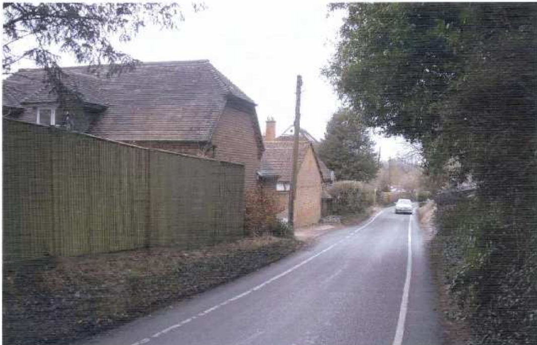
View of existing garage and cottage buildings looking northwards along Village Street.
